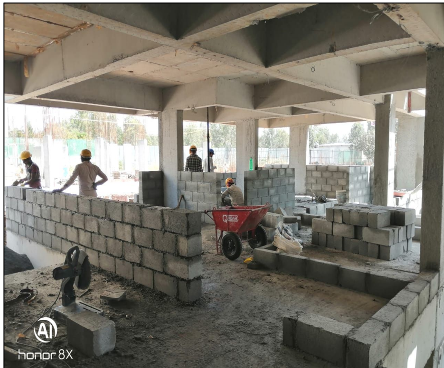
A Block Ground Floor Block Work
