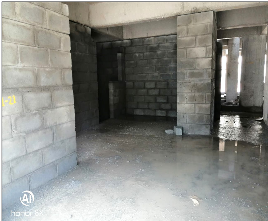
B Wing Ground floor Block Work
