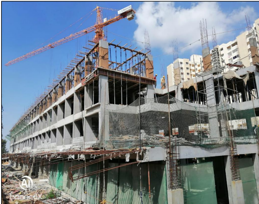
A Wing - Second Roof Beam Shuttering
